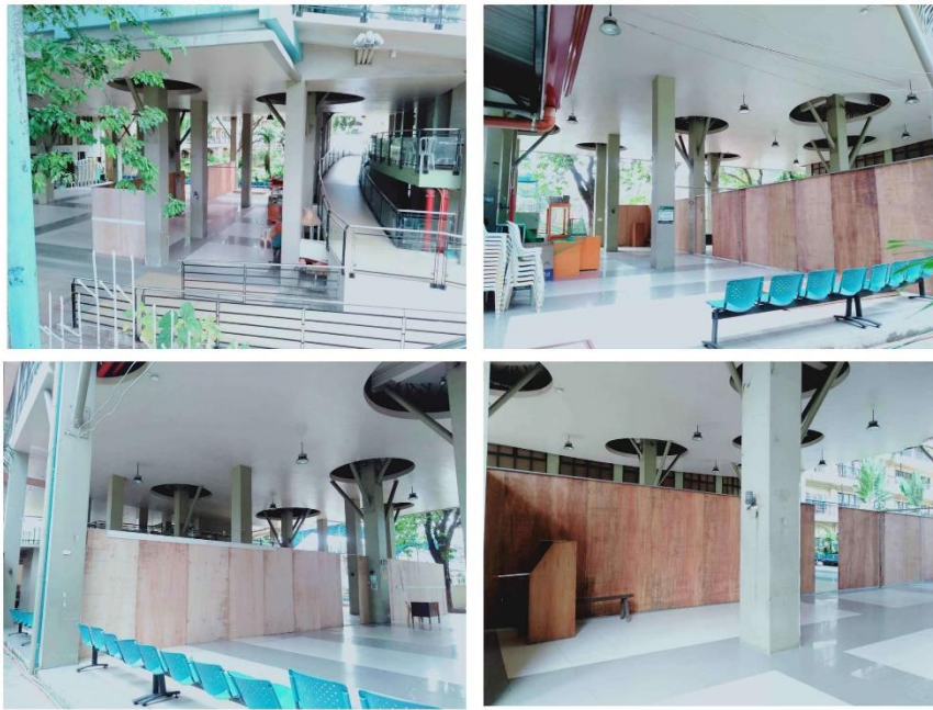
TAC BUILDING (GENDA PER.) EXISTING PHOTOS SCALE
